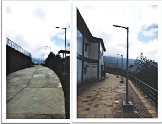
Installation of LED fitting street light
