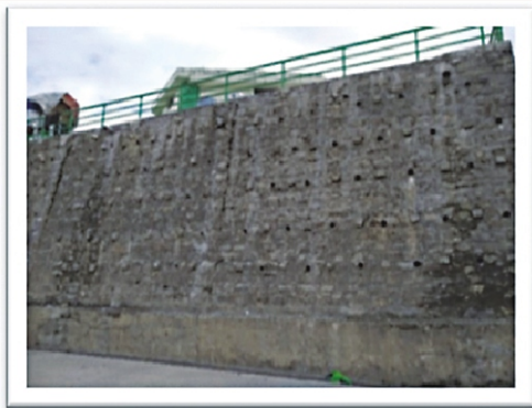
(a) Reconstruction of retaining wall
